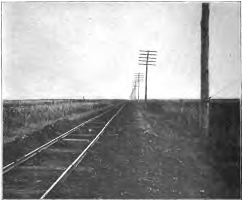
Manner of filling on Belleville turnpike, Bergen Co. This is the second section near the railroad track, about one mile below the starting point.
